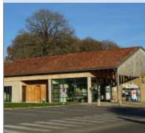
Centre multiservice, St-Pardoux (atopia)
